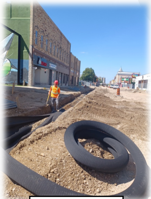
Installation of new roadway subdrains
